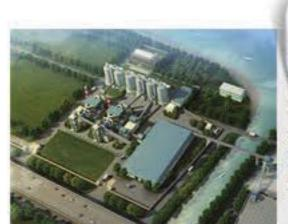
1.5 Million t/a GGBS Plant of Baosteel... It is a two-purpose Production Line with two parts. One is a steel slag production line with annual capacity of 300,000 million tons slag powder ...
