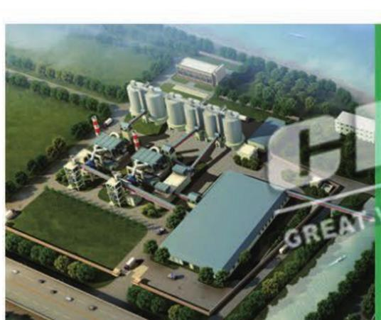
**GGBFS** Grinding Plant innual industrial slag project for Shanghal Bao Steel 1500,000 tons annual Equipment List: belt conveyors, 2GRMS46.41 slag vertical mill, steel slag ball mill, bucket elevator, dust catcher, final
